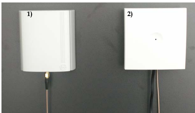
Figure 12 Repeater and External Antenna Installed on the Wall
